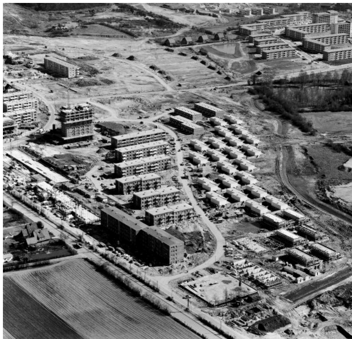
Lohbrügge-Nord in Bau, 1966
